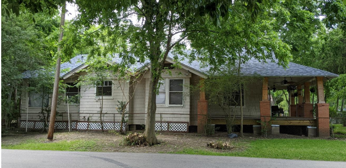
SIDE FAÇADE FACING HILLSBORO STREET PHOTOS BY PRESERVATION HOUSTON
